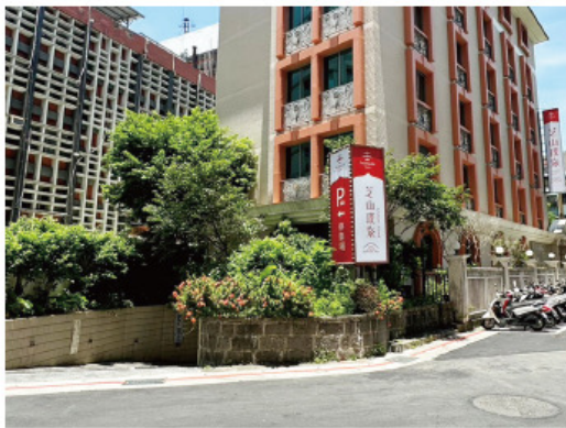
Underground Parking Lot
